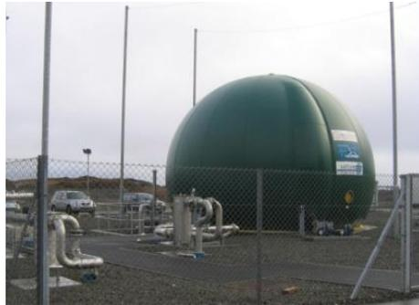
Figure 2 – Example of Biogas storage system
