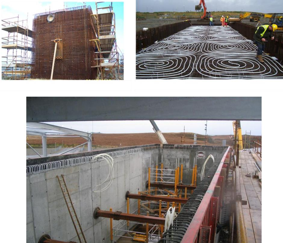
Figure 3. CREED biogas digester being built
