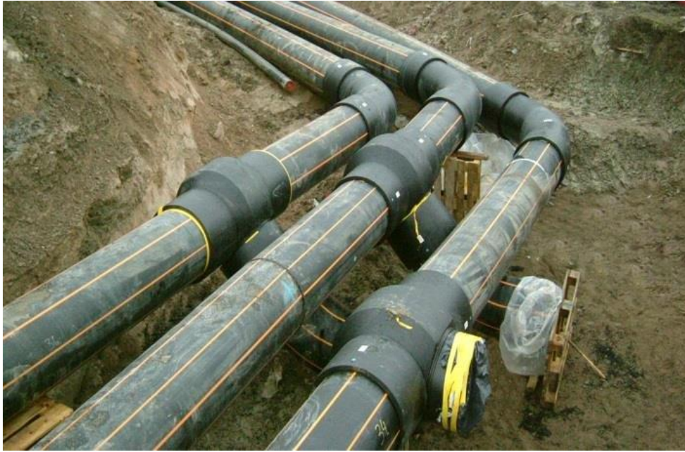
Figure 9.1 - Polyethylene pipelines used to distribute natural gas 24
