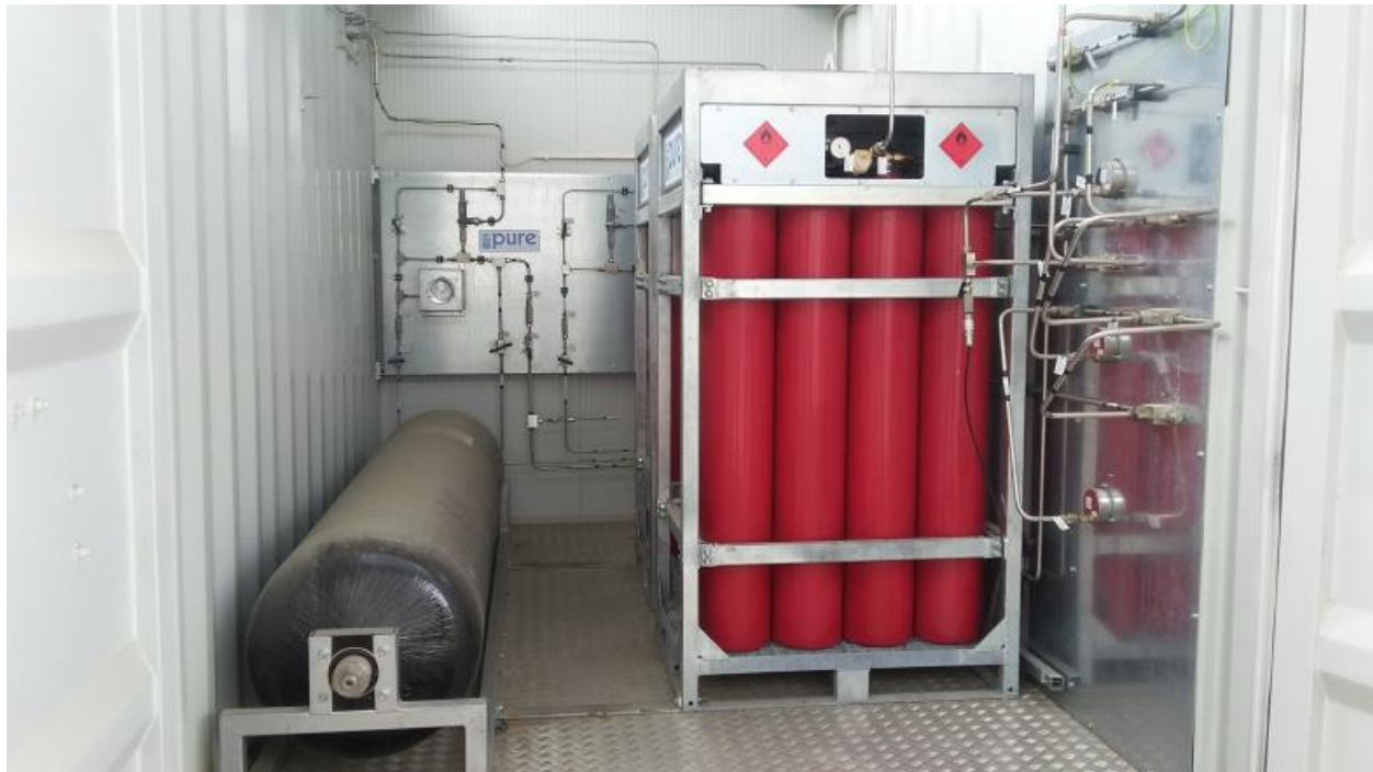
Figure 2.1 – Compressed gas storage – Composite (left), MCP (right) 1
